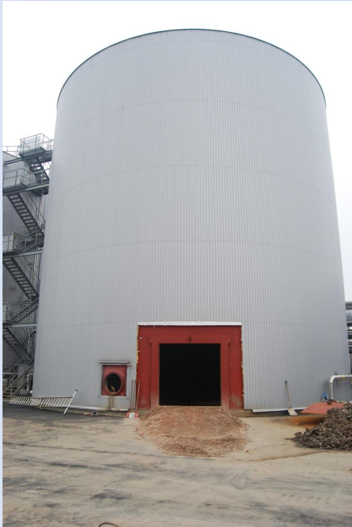
manhole and entrance for machine
