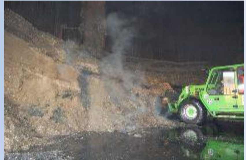
Sand-digging with a wheel loader
